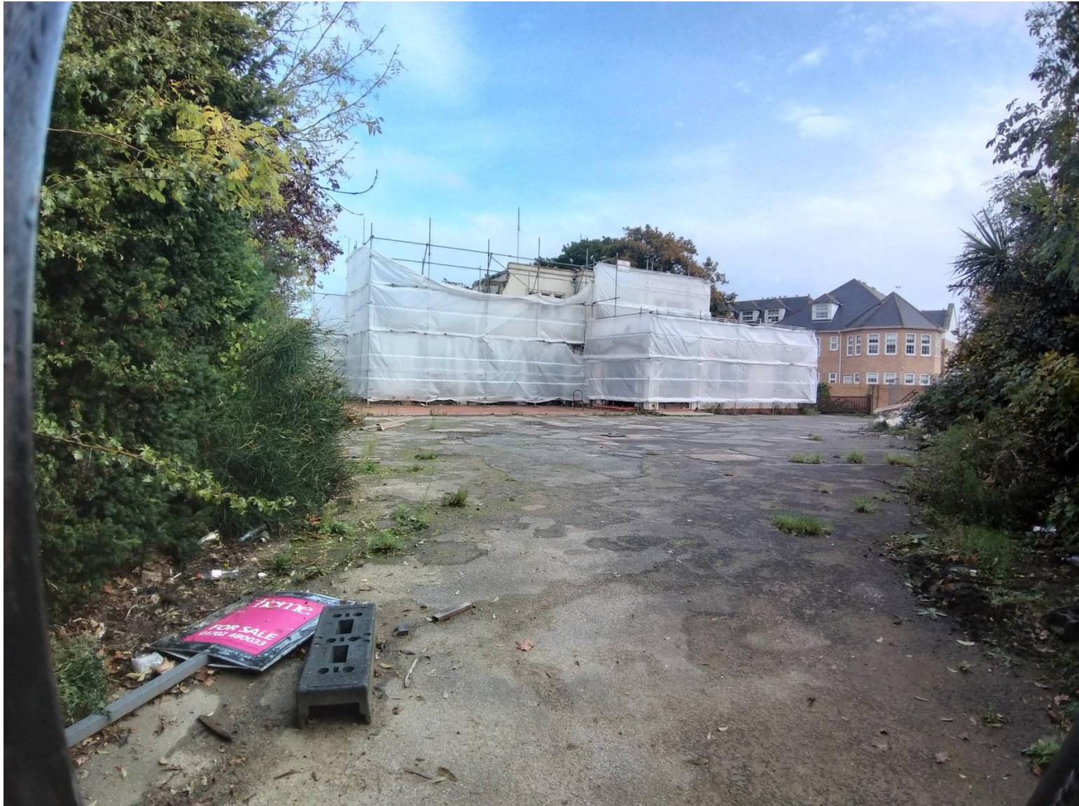
The derelict building on site
